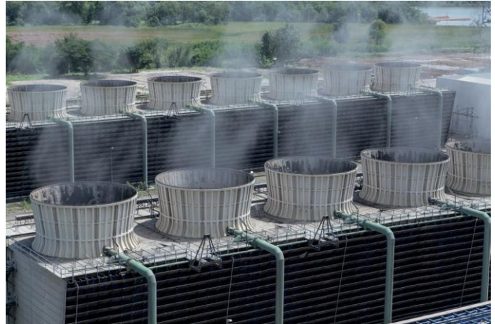
Typical open cooling towers
